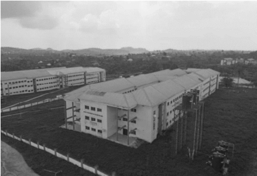
Figure 7 | An aerial view of the Awosika Hostel Source | The Directorate of Physical Planning, FUTA.
